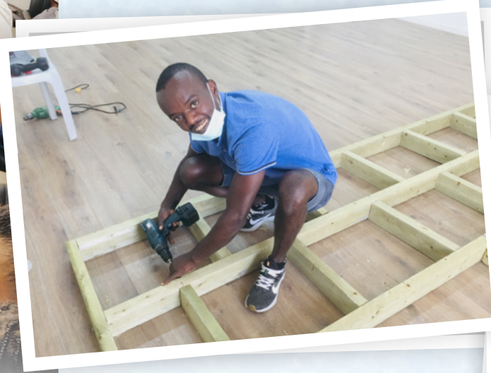
Stefanos building the stage in Beresheet's newest meeting place
